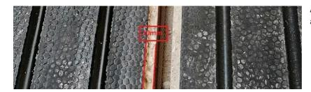
After unrolling, align the flooring with a distance of approx. 10 mm to the gutter.
