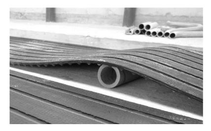
**Expert Tip:** To reduce friction between the continuous rubber flooring and the concrete, place rollers underneath every 3 m. This helps distribute the tension evenly along the entire length of the flooring.
