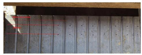
Secure two rows of A2 10x80 nail-in anchors. First row approx. 50 mm from the edge of the rubber flooring.
