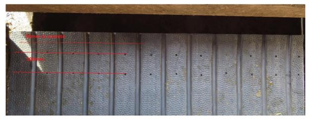
Secure two rows of 10x80 nail-in anchors. Drill  $\emptyset$  11mm holes in the tread bars, just as done for the first short side. The first row should be positioned 50mm from the edge of the flooring, with the second row approximately 100mm further in
