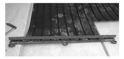
Attach a suitable tensioning device that distributes the applied tension evenly across the entire width of the flooring (e.g., two metal rails screwed together). Then, tension the flooring by 1.5%, for example using chain hoists.
