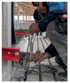
The cover sheet must be prestressed by 1-1.5 % (1 % corresponds to 10 cm per 10 m). The tensioning device should distribute the exerted tension over the whole width on the cover sheet. For example, use 2 rails (one on the top side, the second on the bottom side of the deck). Chain hoists or tension belts can be used for tensioning.
