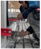
Tension the cover sheet by 1–1.5 % (1 % corresponds to 10 cm per 10 m). The tensioning device must distribute the load evenly across the width of the cover sheet. For example, use two rails — one on top, one underneath — and apply tension using chain hoists or tensioning straps.
